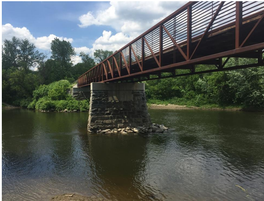
Figure 3 LVRT Bridge 68 in Jeffersonville
