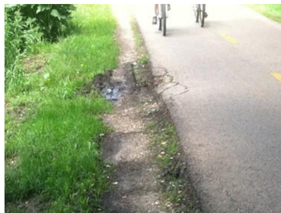
Figure 41. Photo. Inadequate shoulders on a path resulting in edge damage (FHWA, 2013a).
