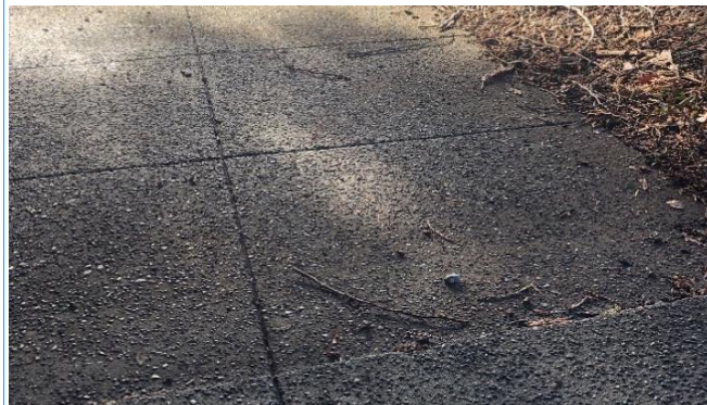
Figure 13. Photo. Example of tensile shrinkage.
