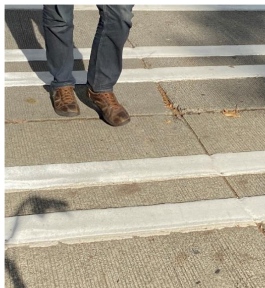
Figure 25. Photo. New thermoplastic markings installed over existing markings can cause accessibility challenges due to depth of the marking reveal.
