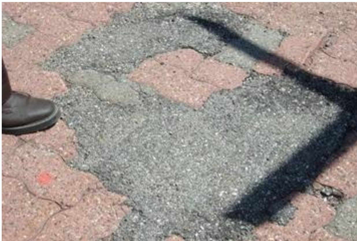
Figure 35. Photo. Damaged pavers have been repaired with asphalt to alleviate a trip/fall risk (FHWA, 2013a).
