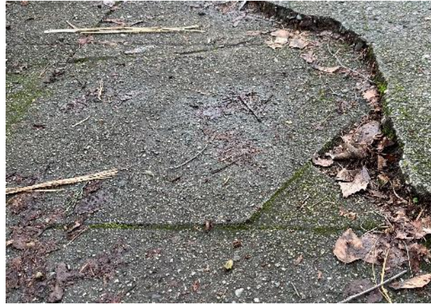
Figure 14. Photo. Example of sagging.
