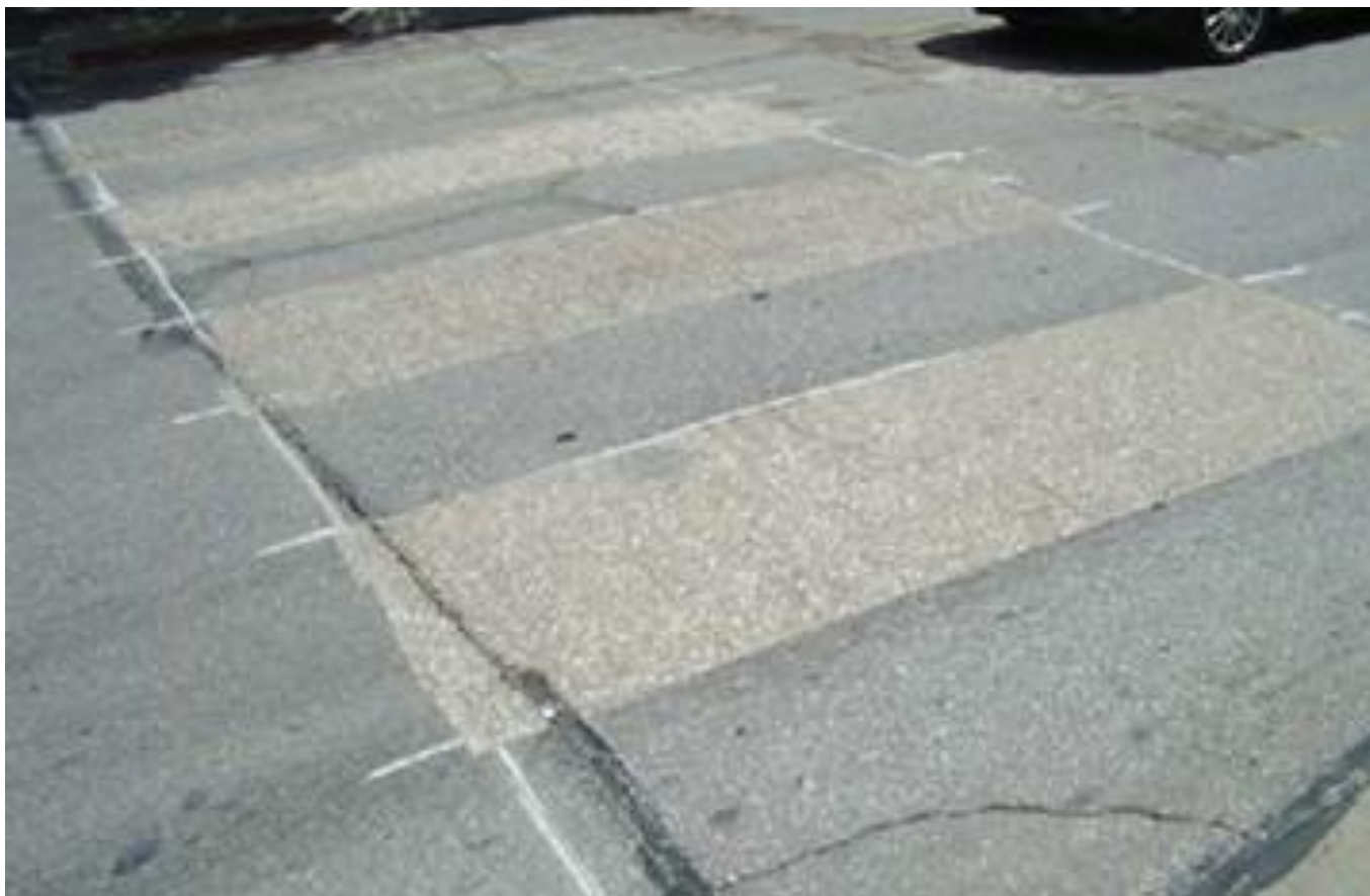
Figure 38. Photo. Old crosswalk markings removed for new crosswalk marking tape (FHWA, 2013a).
