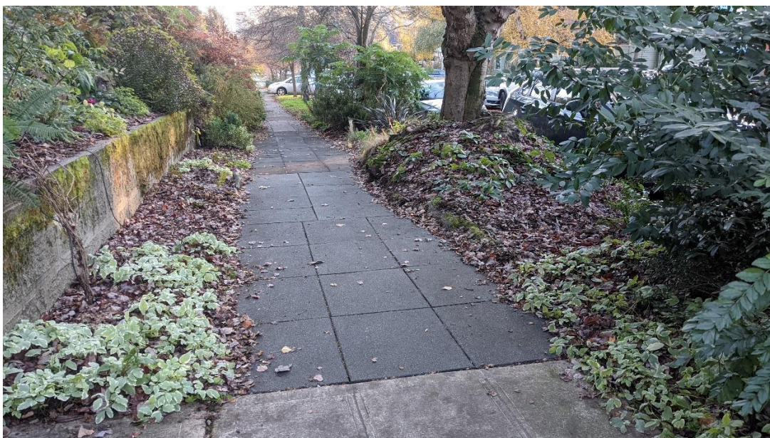
Figure 37. Photo. Rubber pavers provide a flexible solution for maintaining accessibility while promoting mature tree health.
