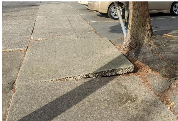
Figure 15. Photo. Example of raised or heaved pavement.
