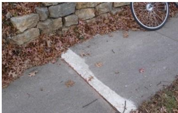
Figure 31. Photo. A raised sidewalk block has been ground down to provide a smoother transition (FHWA, 2013a).
