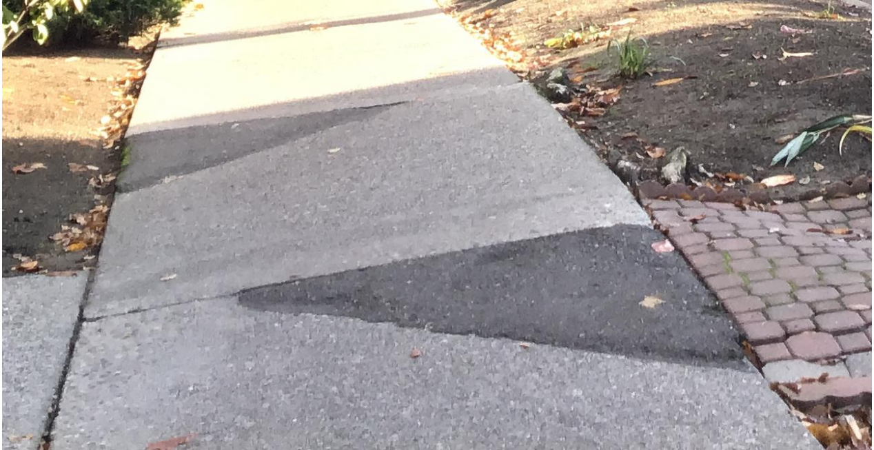
Figure 21. Photo. Temporary asphalt wedging.
