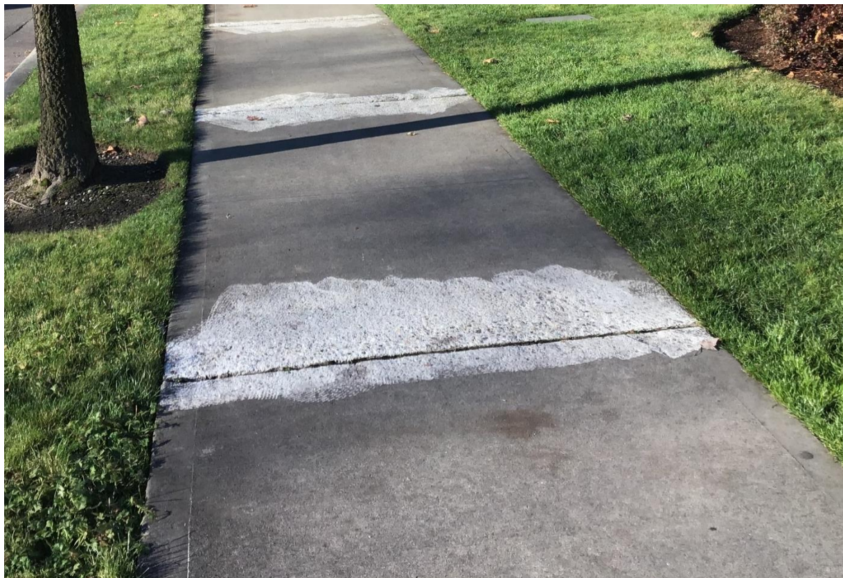
Figure 24. Photo. Grinding or horizontal cutting is a low-cost maintenance method that can address accessibility barriers and extend the life of a sidewalk if done properly.
