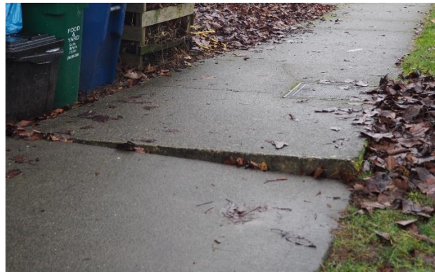
Figure 12. Photo. Example of a rigid body uplift or settlement.
