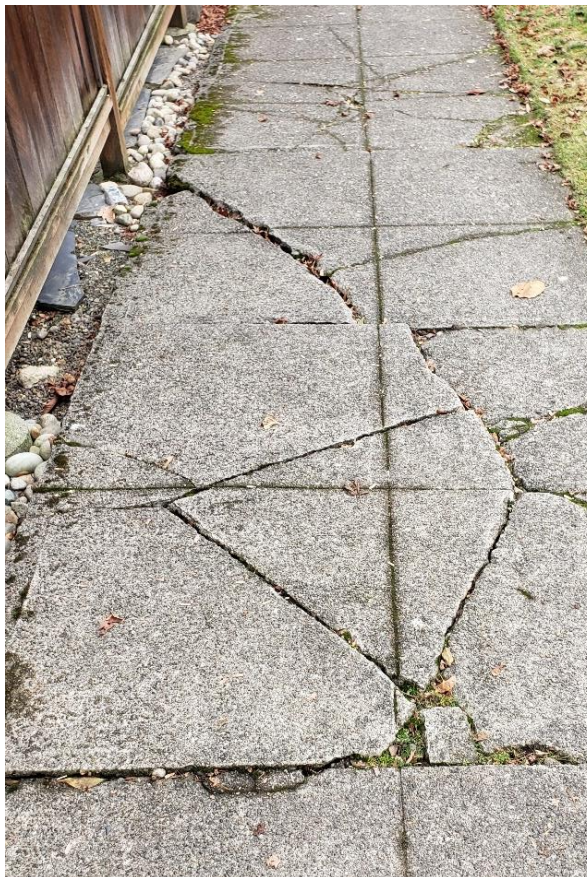
Figure 16. Photo. Example of cracking.
