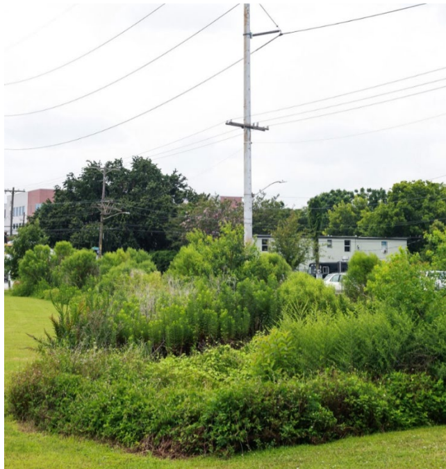
Figure 8. Example bioswale along the Lafitte Greenway in New Orleans, Louisiana. Image source: Friends of Lafitte Greenway
